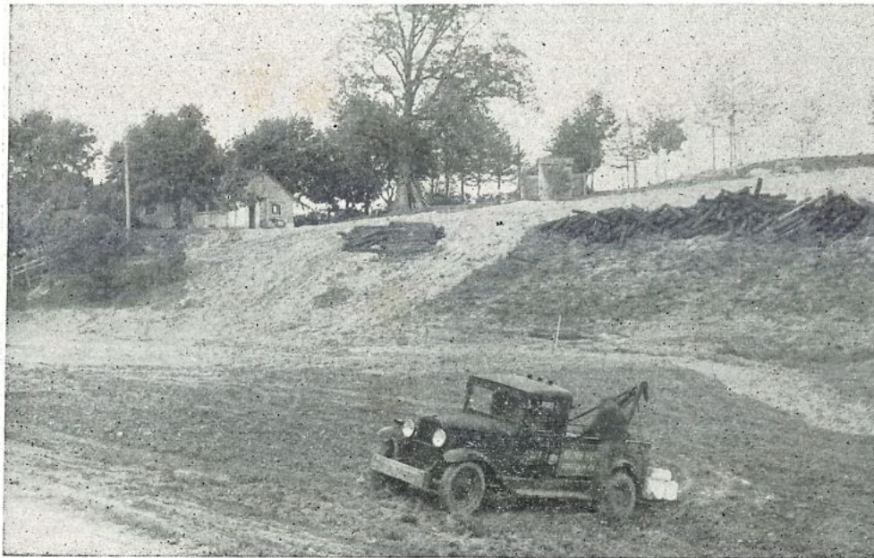
GETTING AMPHITHEATER OUT OF DIRT
