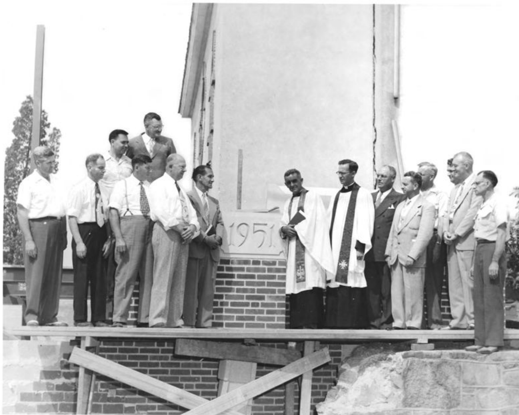
Cornerstone laying – August 19, 1951. Photo by Owen C. Stout.
