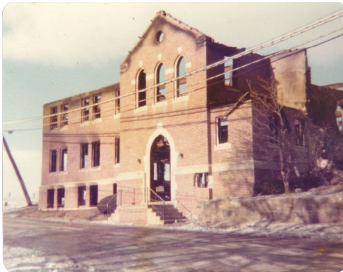
Above & Below: Before the walls of the Sunday School building were knocked down.
