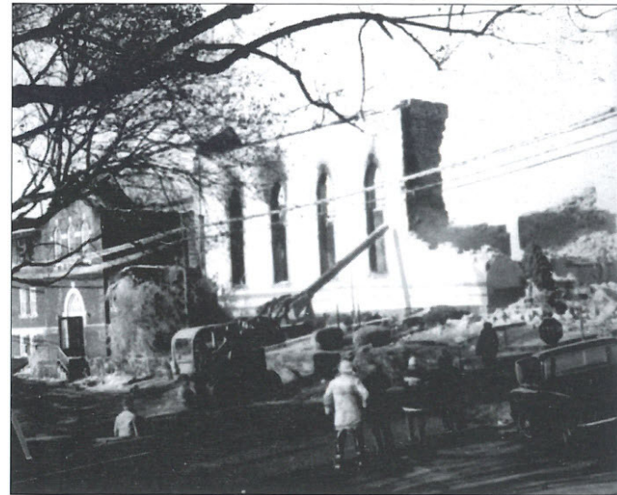
Above & Below: Heavy equipment knocks down walls of the church and Sunday School building.
