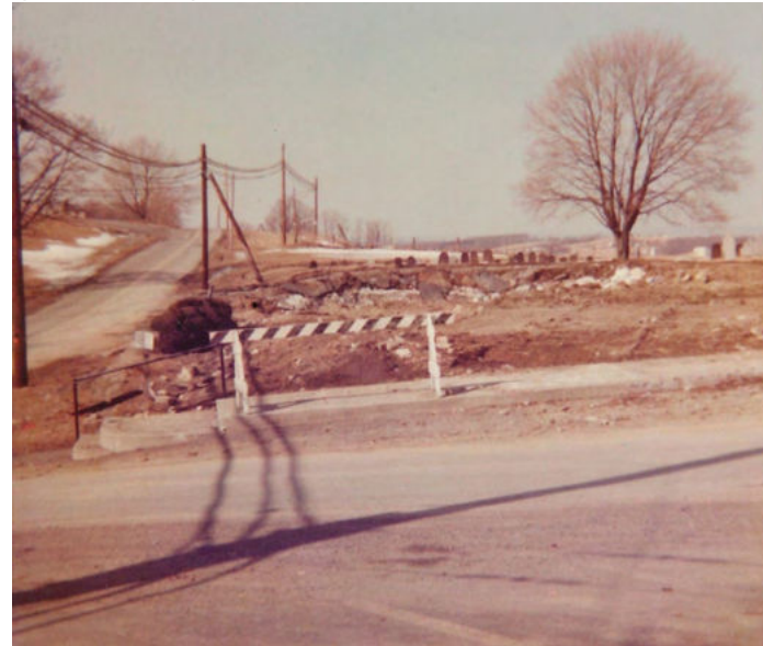
The former church site has been cleared.
