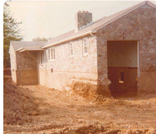
The foundation is dug out and prepared. Above photo: Joyce Hassler
