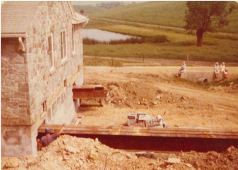
Steel beams are removed after the move. Above photo: Nancy Wolfskill
