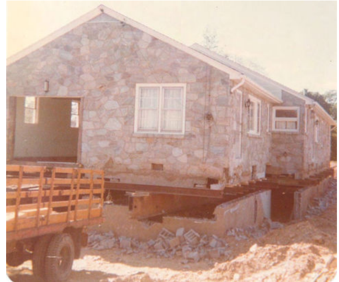
Steel beams are placed under the house. Above photos: Joyce Hassler
