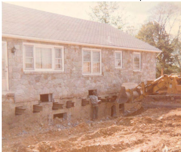
Steel beams are placed under the house. Above photo: Joyce Hassler
