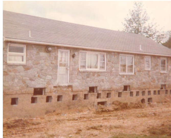
The foundation is dug out and prepared. Above photos: Joyce Hassler
