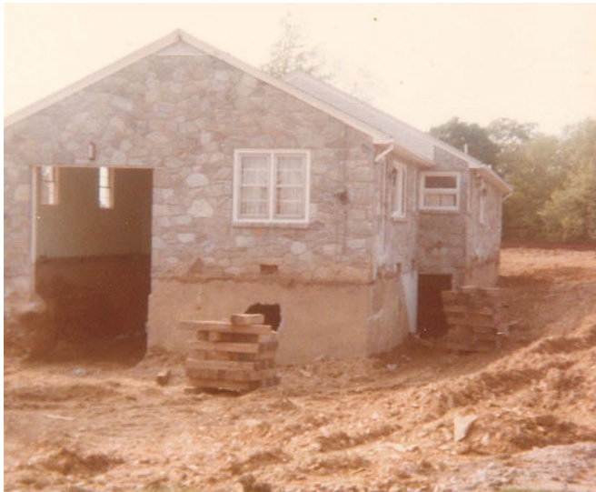
The foundation is dug out and prepared. Above photos: Joyce Hassler
