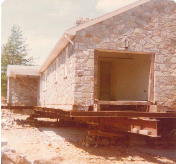
Steel beams are placed under the house. Above photos: Joyce Hassler
