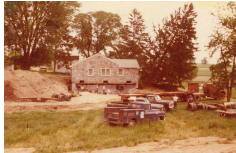
New foundation in progress. Above photo: Nancy Wolfskill
