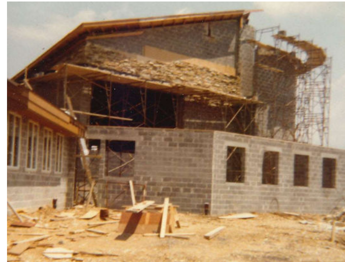
Drystack stone on left side of Chi Rho wall June 25, 1978 – Marge Baerncopf photo
