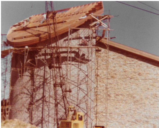
Roof of Chi Rho wall under construction – undated photo
