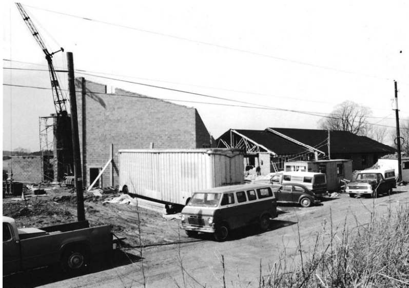
Construction continues – March 1978
