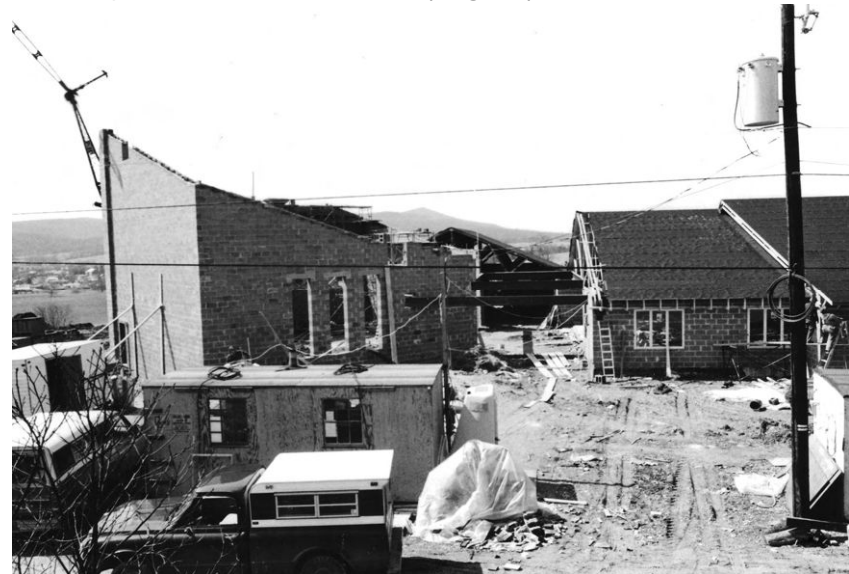
Construction of Sanctuary and Narthex – March 1978
