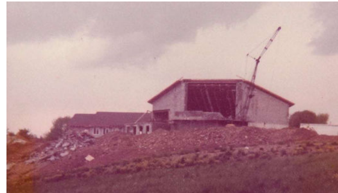
Chi Rho wall under construction – Spring 1978
