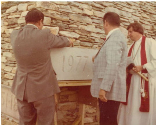
Mark Wolfskill and Vernon Bright place the groundbreaking program and the church constitution in the cornerstone, with Pastor Cloughen
